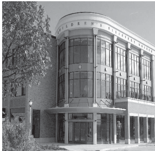
The Children's Discovery Museum in Normal was designed by local Francois Associates Architects.
